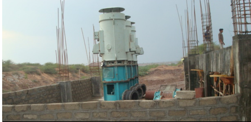
View of Jackwell-cum-Pump House of Rajankollur LIS
