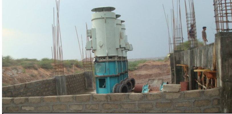
View of Jackwell-cum-Pump House of Rajankollur LIS
